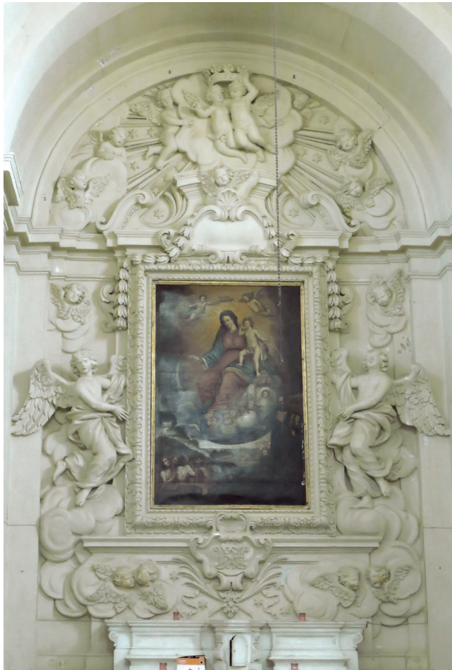
Fig. 9 The altar reredos before restoration. (Photo: Restoration and Preservation Department, Malta)
